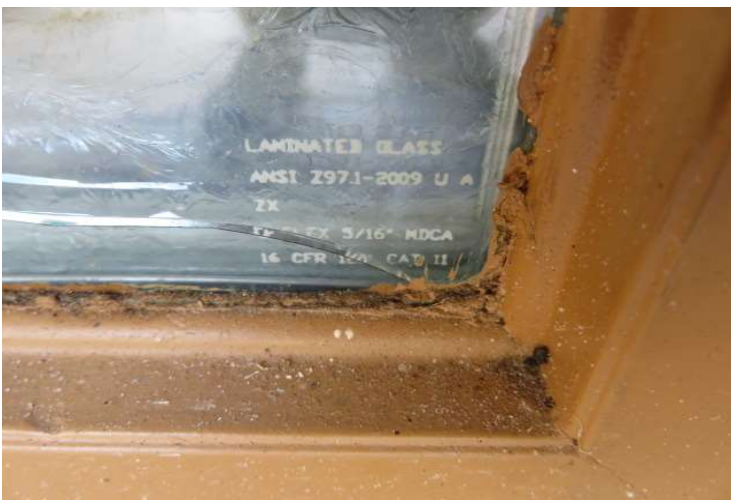
All other openings are glazed and all are impact rated - LAMINATED GLASS - MDCA -
